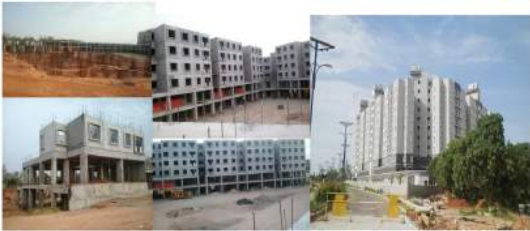
Construction of Aspen Block for Ms. Brigade Orchards
