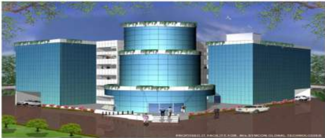
Construction of IT Facility Park of 1Lakh Square foot at KIADB Industrial Area, Bommasandra , Bangalore.
